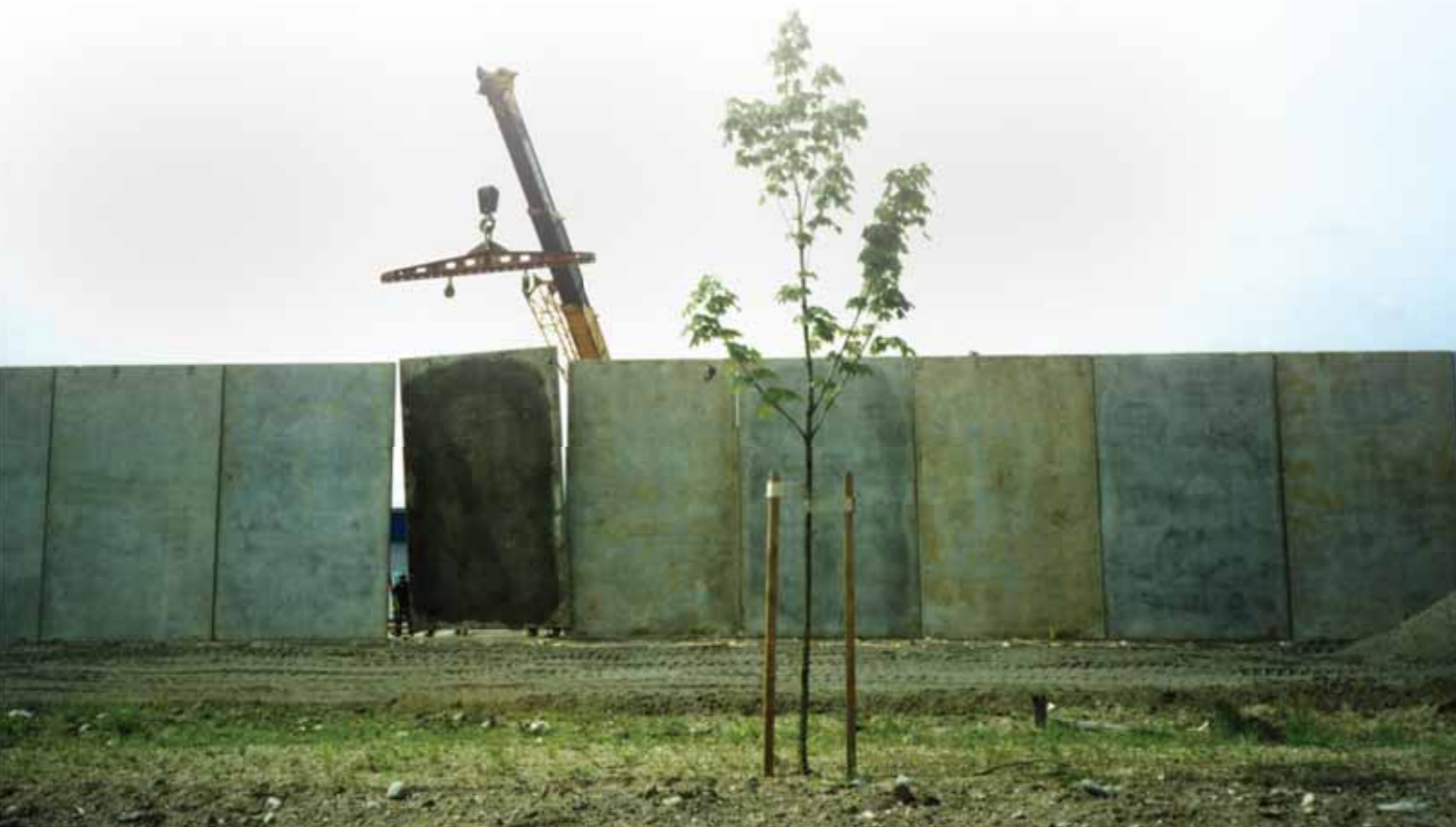
A final “closure” panel is hoisted into place.
