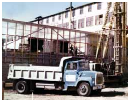
FROM TOP: Part of the Parker Street property was converted into artists' studios and Beedie Construction built a new 100,000-square-foot facility that was leased to Barber-Ellis. Main floor plan of the Parker Street building.
