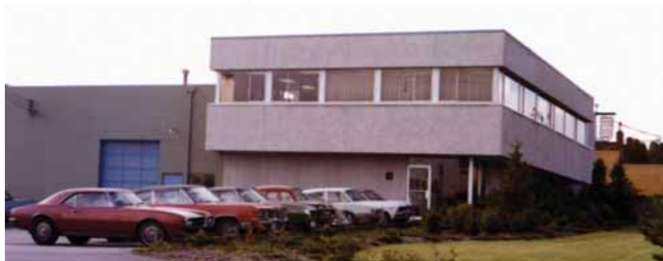
An elevation drawing and photograph of the Alcan building at 3454 Lougheed Highway, completed in 1970.
