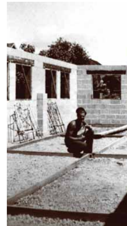
Laying screens for the concrete floor of the Marpole workshop.
