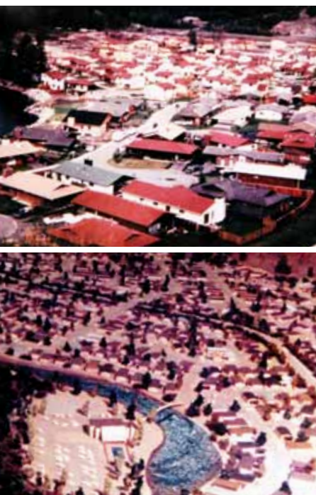
FROM TOP: An aerial shot of a neighbourhood in River Springs in the 1980s. A sales model of the River Springs project.
