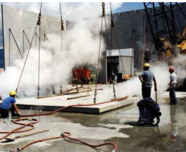
Getting a tilt-up panel ready at a Beedie work site. Keith was always learning as much as he could about new building techniques. When tilt-up construction caught on in the U.S., he went down to find out more. A problem with poor bondbreaker required steam to loosen the panels on this job.
