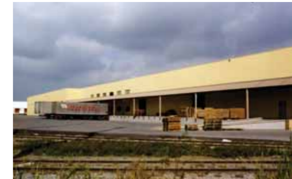
The Schenker warehouse that Beedie Construction built on the Richmond property acquired from BC Hydro.
