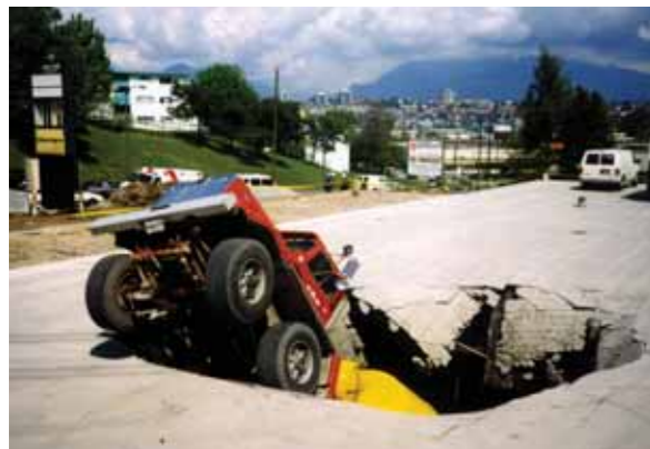
FROM TOP: While some repair work on the parking lot was underway, a cement truck driver ignored the cars-only warning sign and drove his fully loaded vehicle onto the lot. The Electrohome parking lot.
