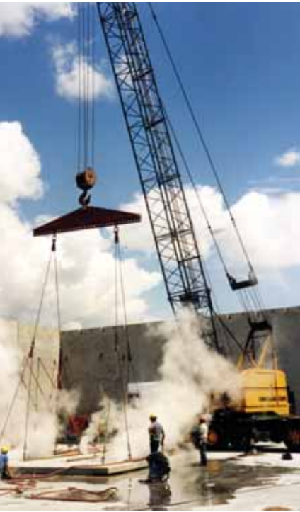
Getting a tilt-up panel ready at a Beedie work site. Keith was always learning as much as he could about new building techniques. When tilt-up construction caught on in the U.S., he went down to find out more. A problem with poor bondbreaker required steam to loosen the panels on this job.
