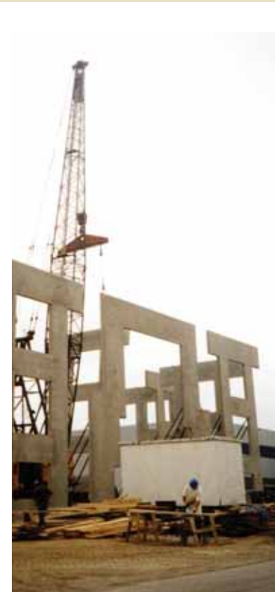
As Beedie projects became larger and client needs more demanding, tilt-up panel designs became more and more complex. The Beedie Group soon became the leading tilt-up specialist in Vancouver.
